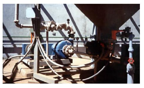
The head of an environmental waste clean-up project in Louisiana described the Discflo system as a "godsend". The pumps, installed in 1994, were used to pump slurry that was dredged from a 23 acre, 50-ft deep site in Lake Charles. The site contained difficult waste products such as hydrocarbons, benzene and many other volatile fluids. The solids content ranges from 2-40%, with viscosities of 20,000 cPs and higher.
